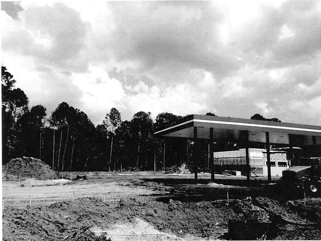
Location for proposed sign on the Northwest canopy face
